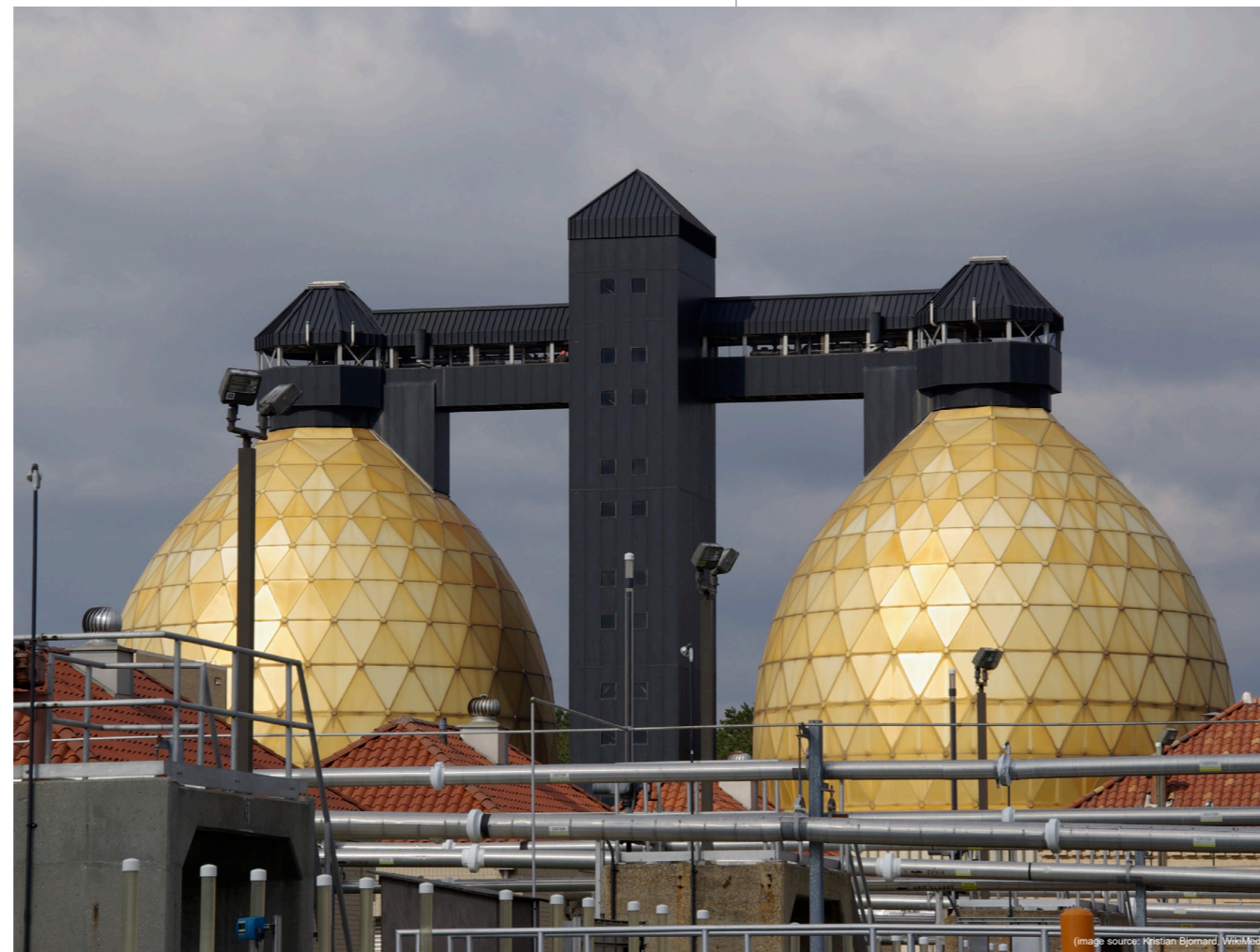
Anaerobic Digesters, Back River WWTW
