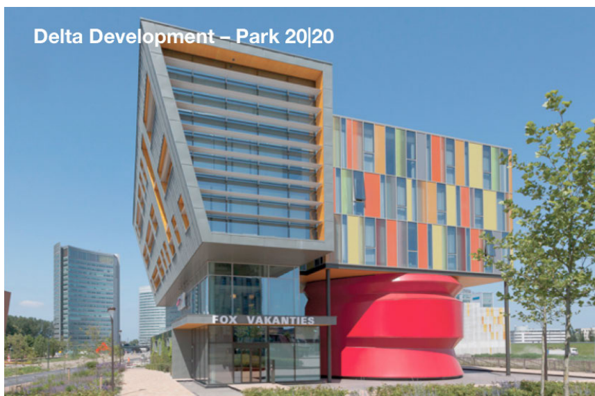
Photo 3: Dutch internet travel booking company Fox Vakanties’ building was the first to receive a BREEAM Excellent environmental rating.
